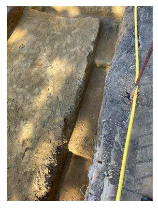
Plates 5, 6. Views of site reduction and stepped foundations
