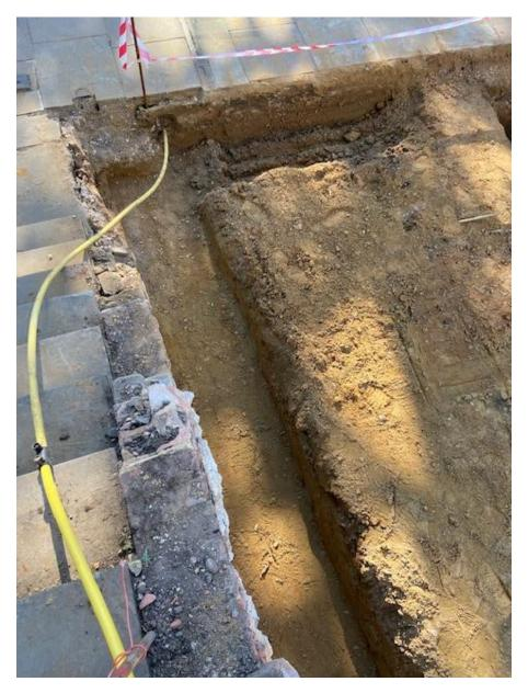
Plate 7. View of site reduction and stepped foundations
